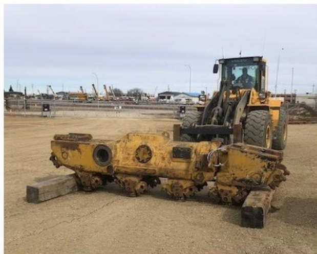
Use the equipment and roll the track frame.
